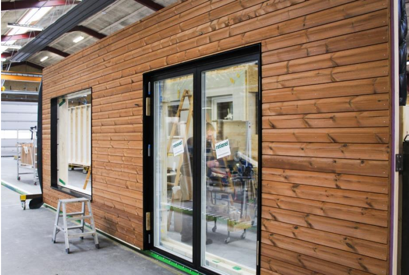
Figure 1: Taasinge Elementer A/S prefabricated facade element (F-2).
