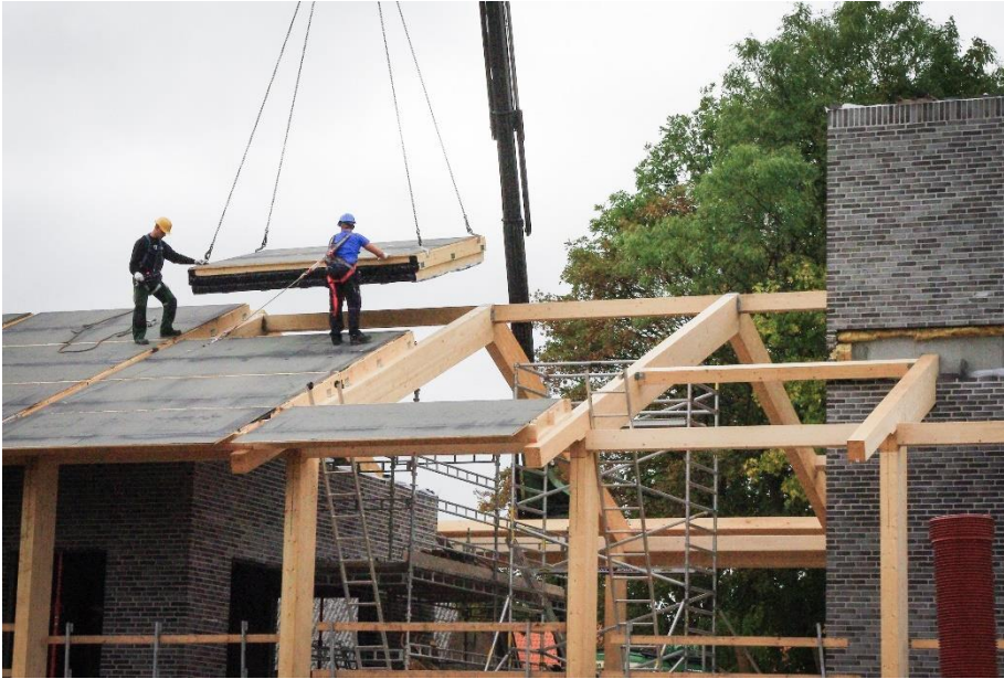
Figure 1: Taasinge Elementer A/S prefabricated roof (T-3a).
